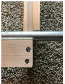
6. Attach 2 spanners stacked on the top side of the head end of the rail leaving 5" at the end. Secure with four 3" screws These double stacked spanners will be used to hold the exercise bar.
